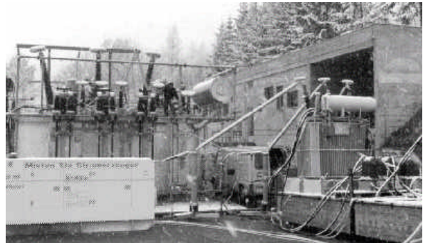
Figure 8: Off-line test set-up for PD-diagnosis on a 220/65-kV transformer using a 350 kVA diesel generator unit (left hand) and a step up transformer 0.4/65 kV (right hand). Transformer under test with torus electrodes at the HV-bushings to avoid corona discharges, and measuring vehicle (background).
